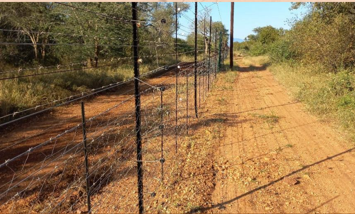
A dangerous game fence (not wildlife friendly) with a combination of wire mesh and electrification
